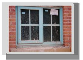
Simply Applied by airless spray or roller, Protectapeel dries and protects windows and frames from construction site damage.
