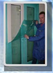
Unlike traditional protection methods Protectapeel contains no adhesives, it simply uses surface tension to bond with the surface, when required it is easily peeled away leaving no residue behind – saving you additional cleaning costs before handover.
