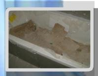
A favorite at Spraylat International, these two pictures show the complete contrast in protection between Protectapeel and traditional film rolls. As you can see the film roll has begun to become unstuck and is letting damaging dust and dirt onto the bath tub. Whereas Protectapeel's skin tight protection has protected the tub during the whole construction project.
