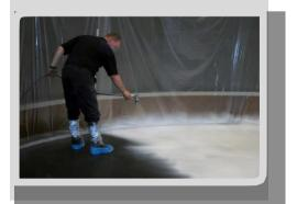
Protectapeel is applied directly to the floor to temporarily protect it from construction site damage. Available in grey as standard or clear or pigmented with a color upon request.
