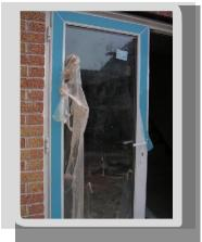
Spraylat do have many construction companies enquiring about Protectapeel after using traditional protective film on rolls. The general consensus is that the traditional films just peel away from the surface during the construction project - as you can see in this image the film has parted from the surface, damaging it causing additional cleaning costs or even worse replacement costs.
